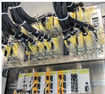
Figure II-9.3 Han® EE and Han® ESS with grip panel
