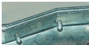
Figure III-2.14 Double labyrinth
